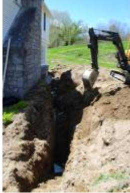
Installing a drainage system Anderson Fred Pierce house.
