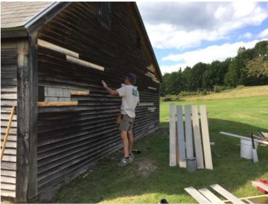
David Brynn replaces clapboards on the Anderson Wells farmhouse.
