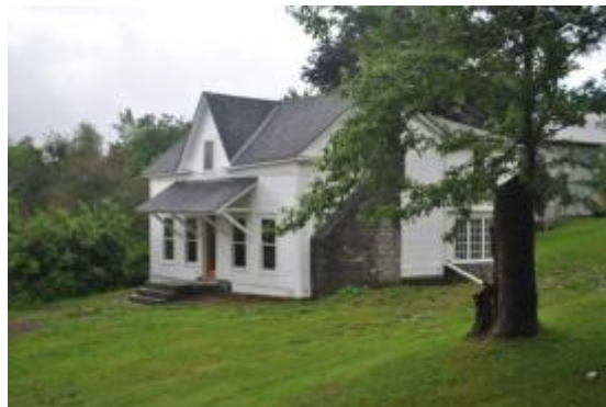
We completed exterior restoration in the summer of 2017.
