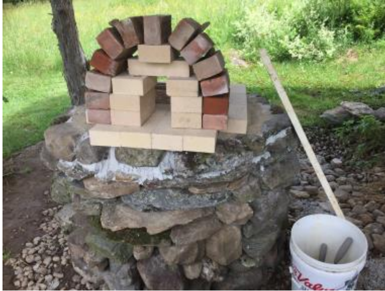
An arch of bricks creates a durable opening for the earth oven.
