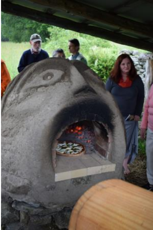
Once the oven was fully fired, we pushed the coals back, swept out the central space on the fire bricks, and slid in the first pizza.
